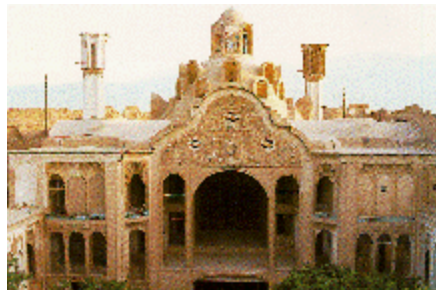
● "Portal of the main portico and the wind towers of Broujerdi House"
